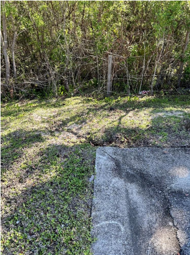
Photo 5. Northeast corner of Moscato Drive dead-end.
