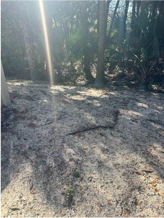
Photo 28, 1507 Verdello Place southwest rear corner.
