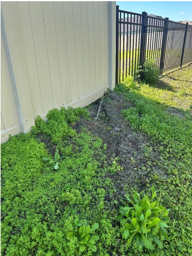
Photo 15, 7734 Fortana Way east rear corner.
