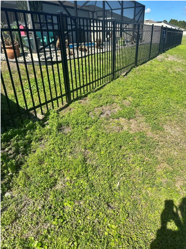
Photo 13, 1330 Moscato Drive rear.
