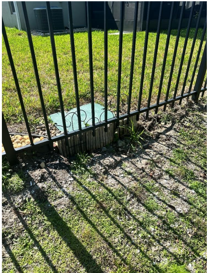
Photo 16, 7704 Fortana Way rear at irrigation box.
