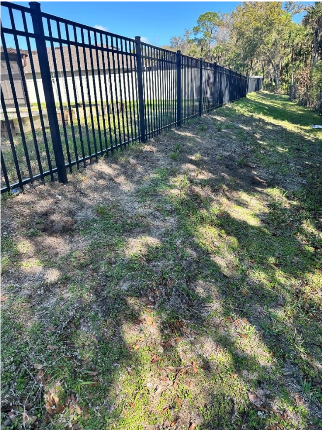
Photo 6. 7691 Prosecco Lane rear.
