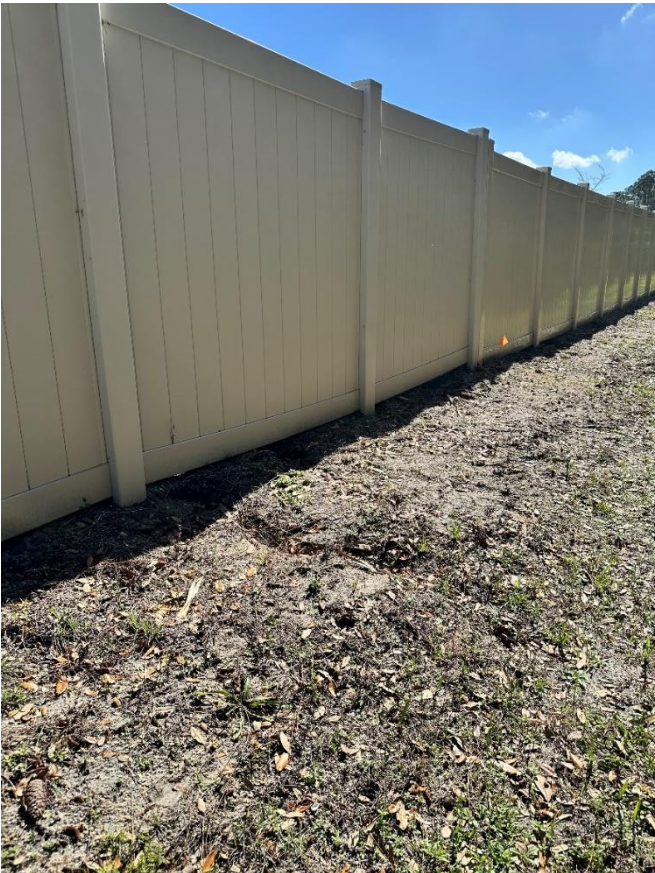
Photo 4, 1389 Moscato Drive rear.
