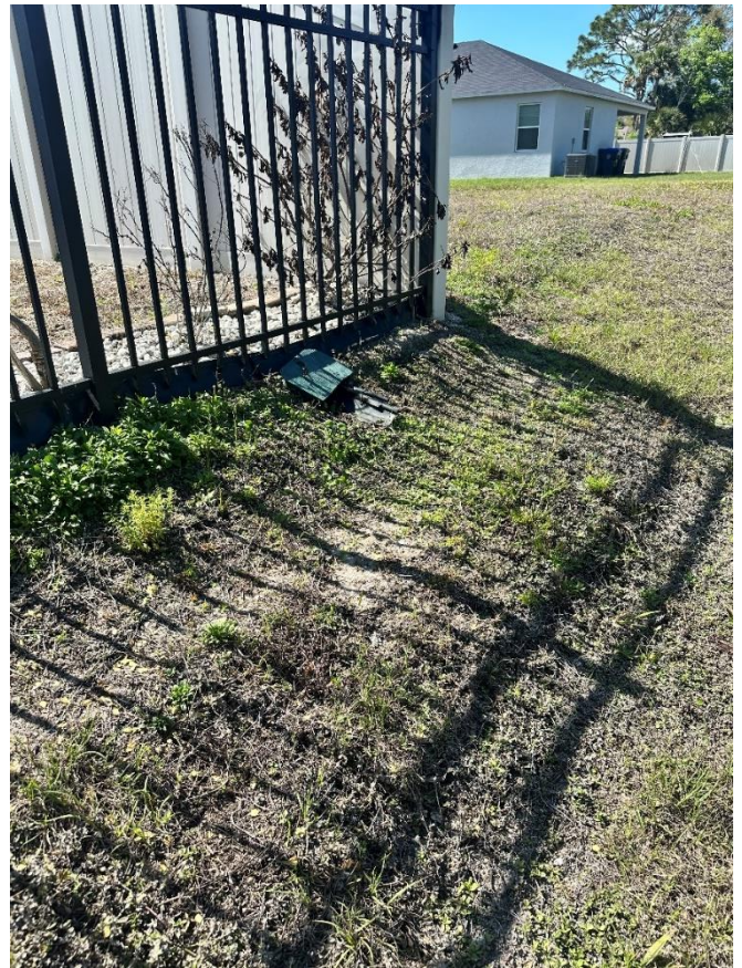
Photo 18, 7694 Fortana Way rear showing piped roof drains.
