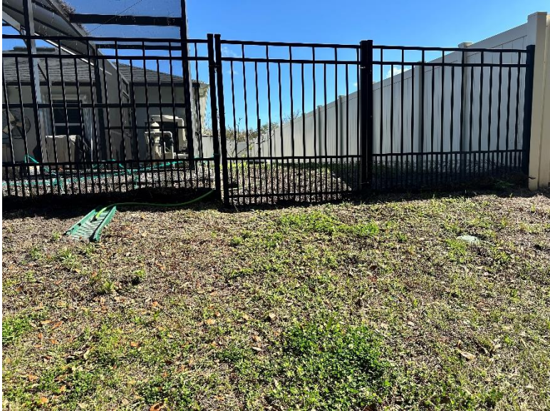
Photo 2, 1399 Moscato Drive east rear corner.
