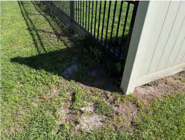
Photo 15. Rear of 1621 Pecorino Court.
