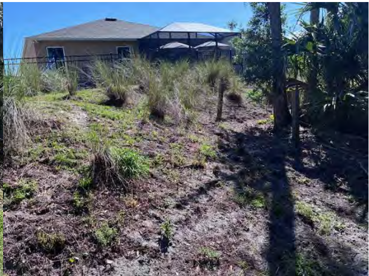
Photo 12. Rear of 1631 Pecorino Court.
