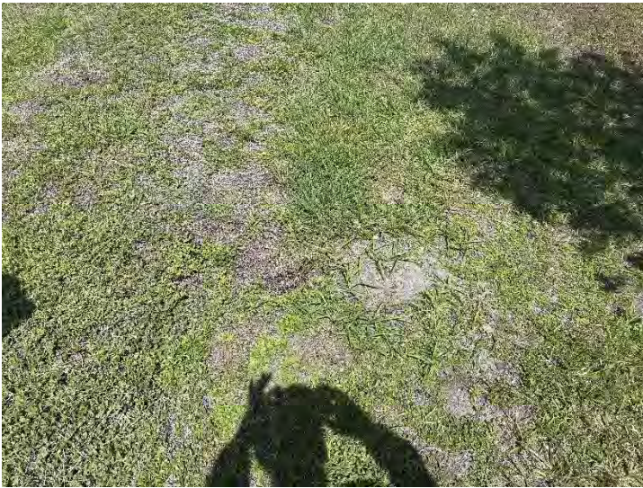
Photo 79. Rear of 1682 Pecorino Court.
