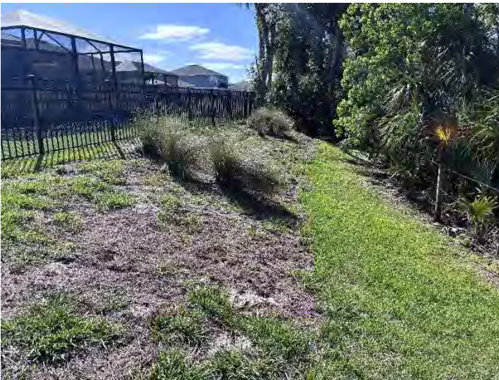
Photo 11. Rear of 1641 Pecorino Court.
