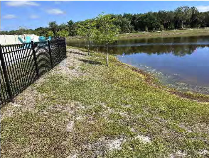
Photo 71. Rear of 1432 Pecorino Court.
